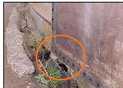
CORROSION HOLES IN THE AST BOTTOM
